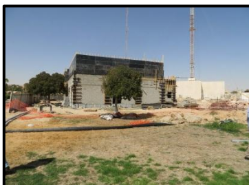
Progress of the Central Arava Medical Center
