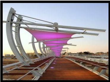
Pipes Bridge in Be'er Sheva
