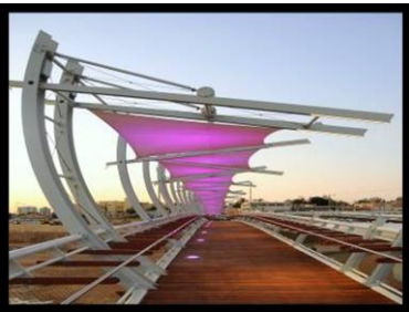
Pipes Bridge in Be'er Sheva
