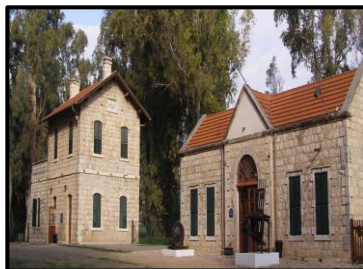
Valley Train Station
