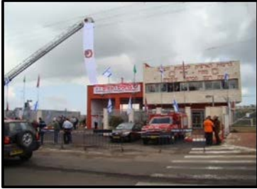
Usafiya Fire Station
